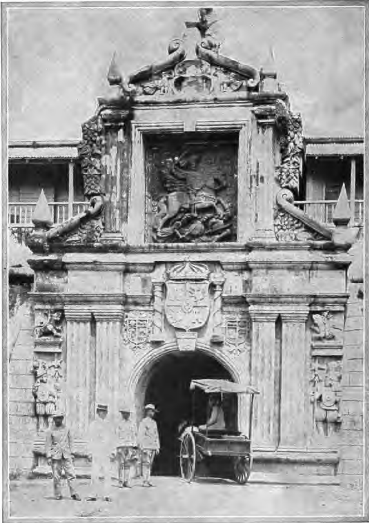
GATE TO FORT SANTIAGO, MANILA.
